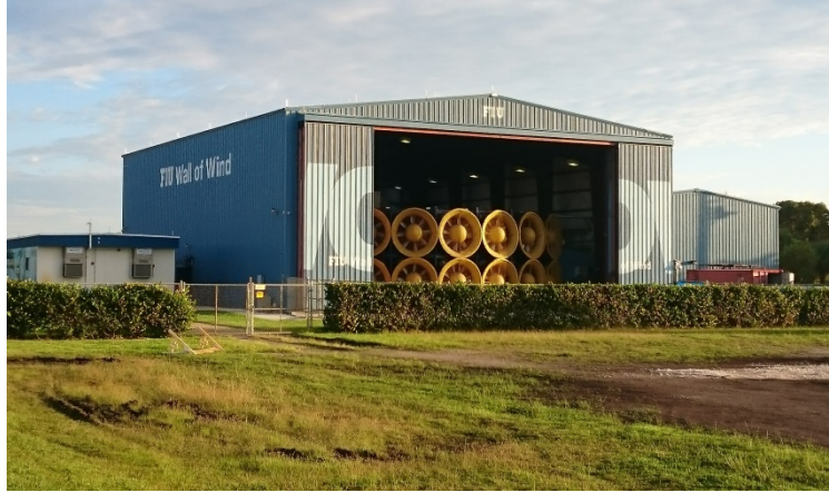
Figure 4-1. The 12-fan Wall of Wind (WOW) facility in Miami, Florida
